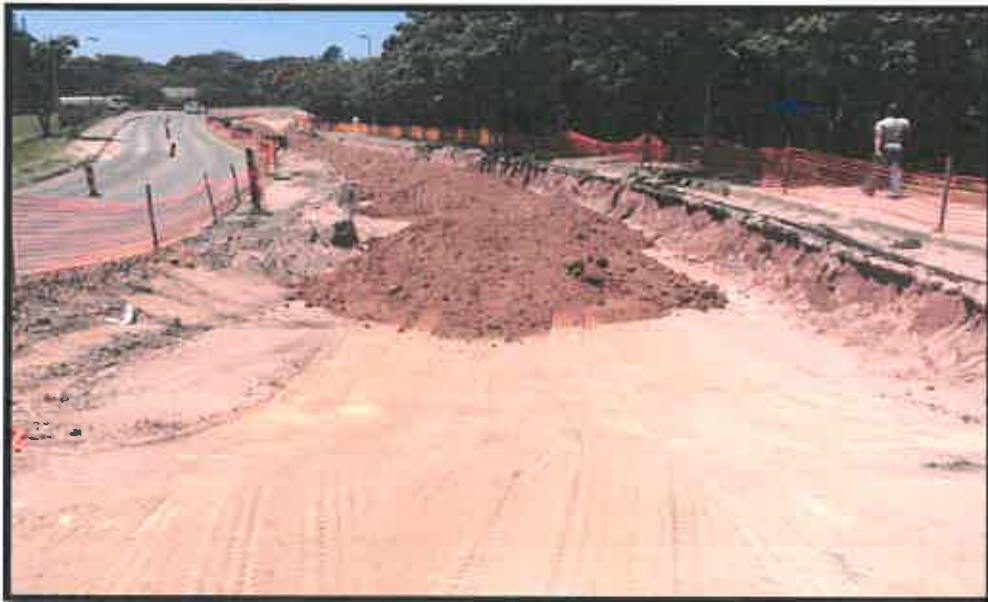
Figure 3: Reconstruction of pavement structure at km 0,65
