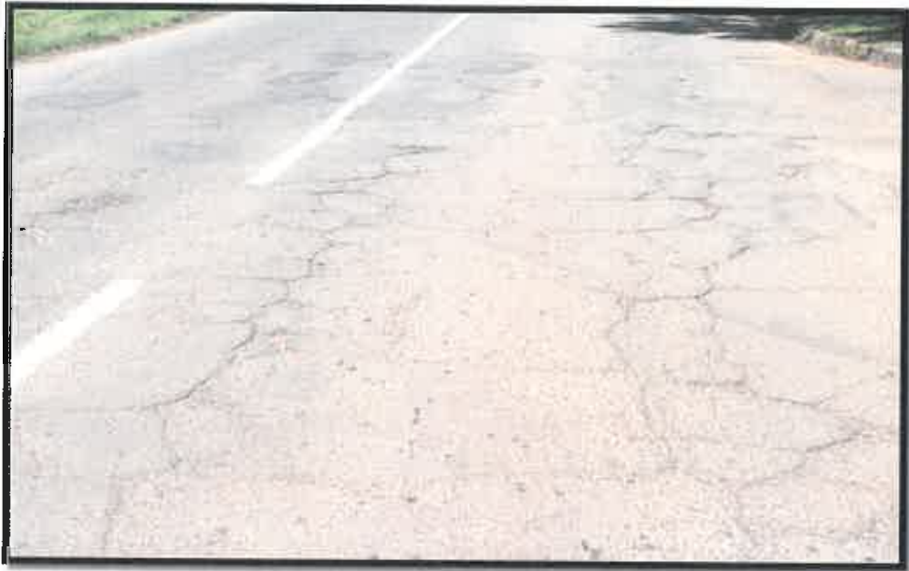
Figure 4: Severe crocodile cracks and patches at km1.65
