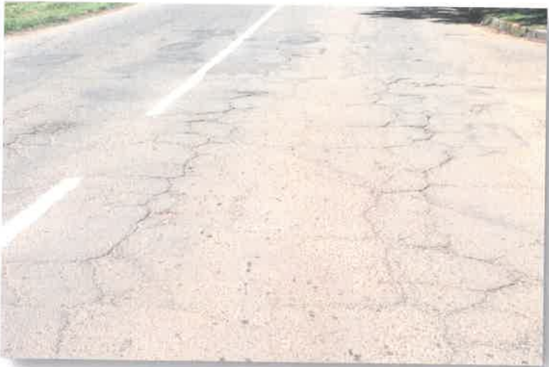
Severe crocodile cracks at KM 3, the section through Eshowe
