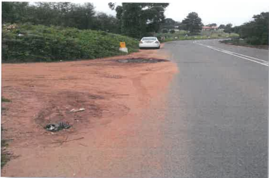
Drainage issues at the bottom of the Super elevation at Km 15
