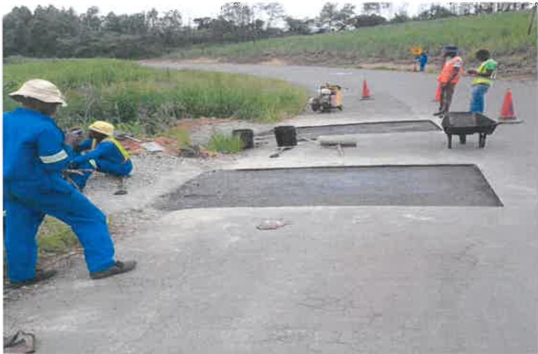
Potholes Repair at Km 22
