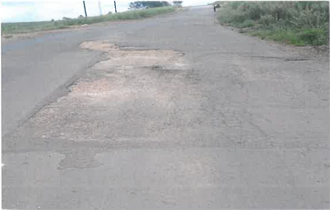
Surface Failure at Km 23
