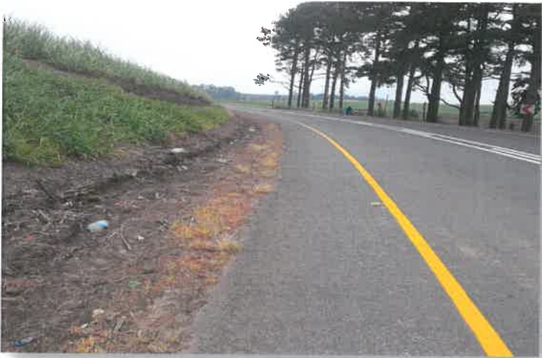
Drainage issues at the bottom of the Super elevation at Km 15
