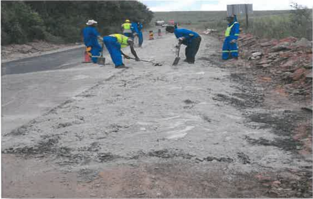
Potholes Repair at Km 22
