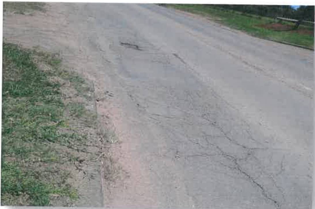
Severe crocodile cracks at KM 3, the section through Eshowe
