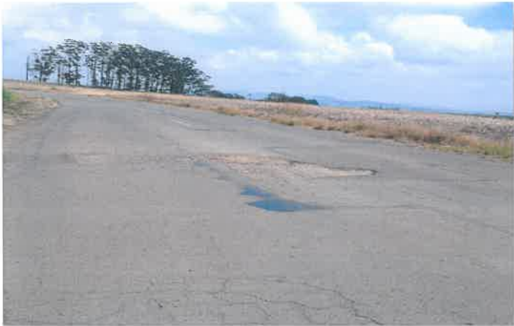
Surface Failure at Km 23
